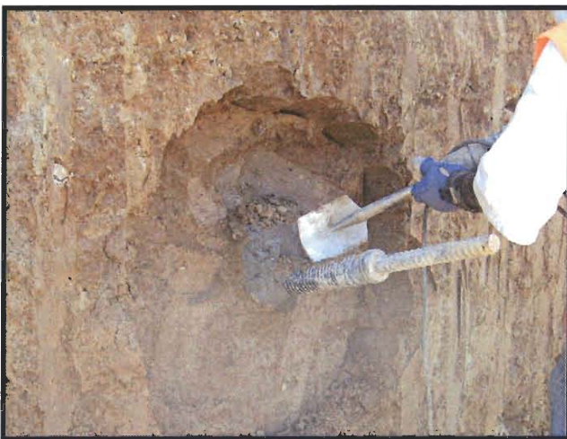
Fig. 10: Recessed Shear Plate
